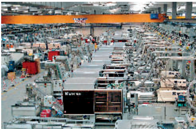
Feeding system for 100 injection moulding machines
