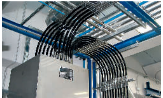
Automatic distribution with ceramic bends
