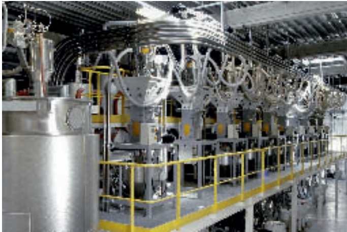
Conveying system of dried and raw materials to gravimetric blenders
